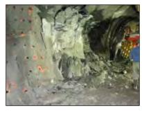
stone, concrete and reinforced concrete. "Dā-mite is mixed with water and placed in the appropriately placed predrilled holes, where it sets and expands, fracturing the rock/concrete". No license required. There are four grades of Dā-mite, providing enough versatility to be utilized in drilled hole diameters from 1 in. to 2 ¾ in.
